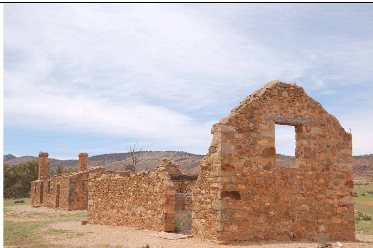
Figure 9: Abandoned Homestead Ruins Near Hawker
