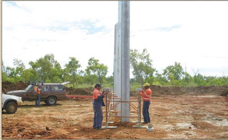
Barkly Highway upgrade, installation of bridge footings and piers.
