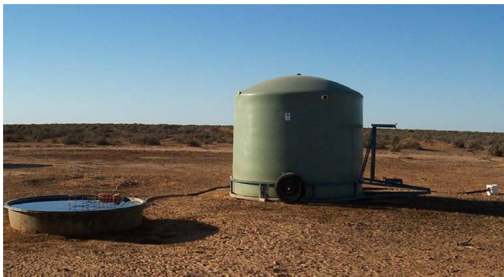
An innovation to make better use of infrastructure has been to use portable tanks that can be moved to different waterpoints. The full costs of infrastructure development were recouped within two years. Image courtesy of Angus Whyte
